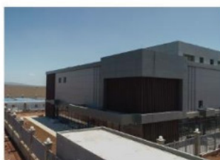
KONZA NATIONAL DATA CENTRE & SMART CITY FACILITIES PROJECT
