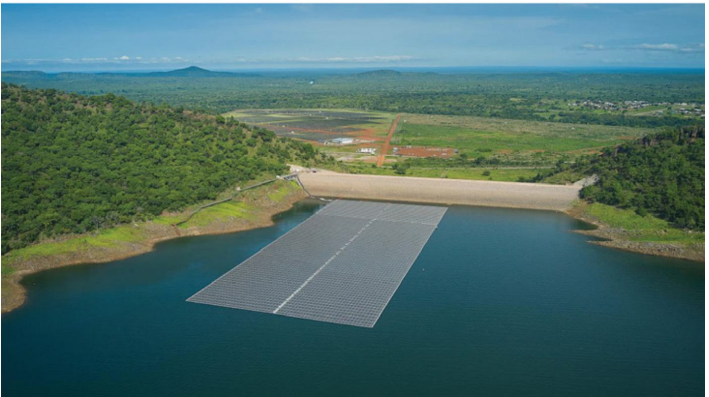
The 1MW Floating Solar at Bui, Eastern Region
