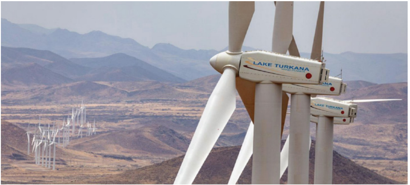
Lake Turkana Wind Power Project
